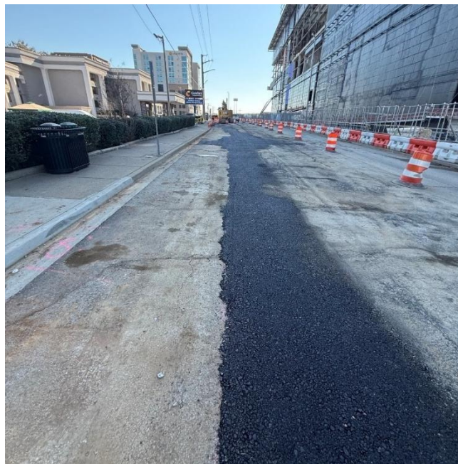
FIGURE 7: INTERSTATE DRIVE SITE PHOTO SHOWING PATCHING OF THE ITS DUCT BANK
