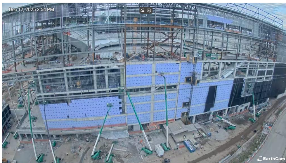
FIGURE 8: SCREENSHOT FROM LIVE CONSTRUCTION CAMERA AT NISSAN STADIUM
