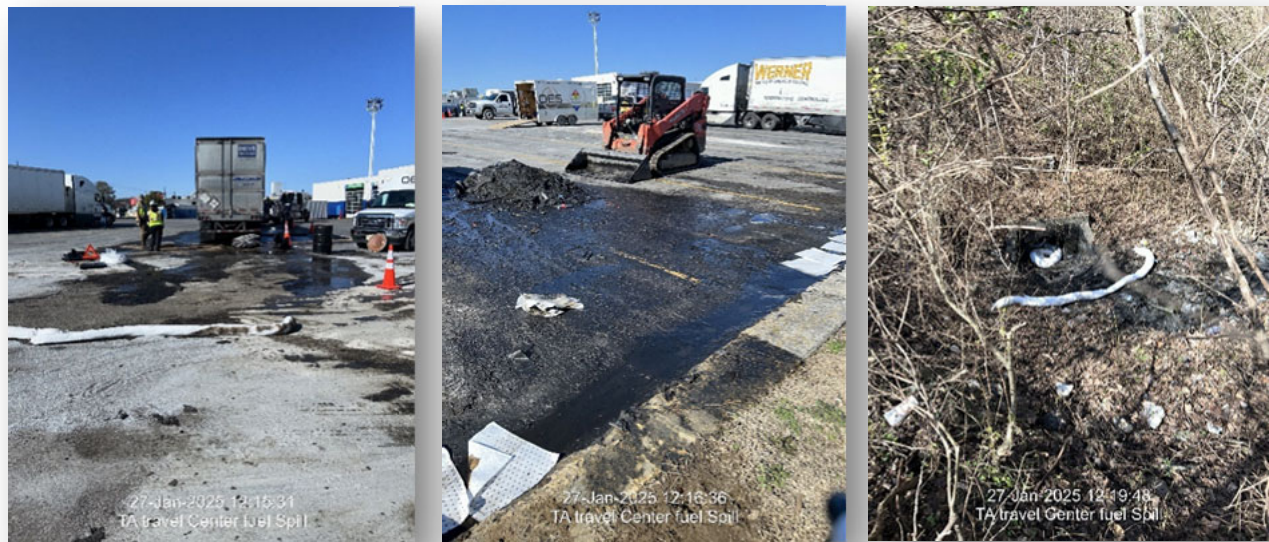
Photos of the Diesel Spill and Old Detention Pond that Contained the Fuel Product
