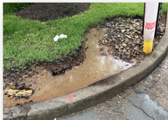
Photos of the Exposed FOG material from Grease Interceptor Overflow
