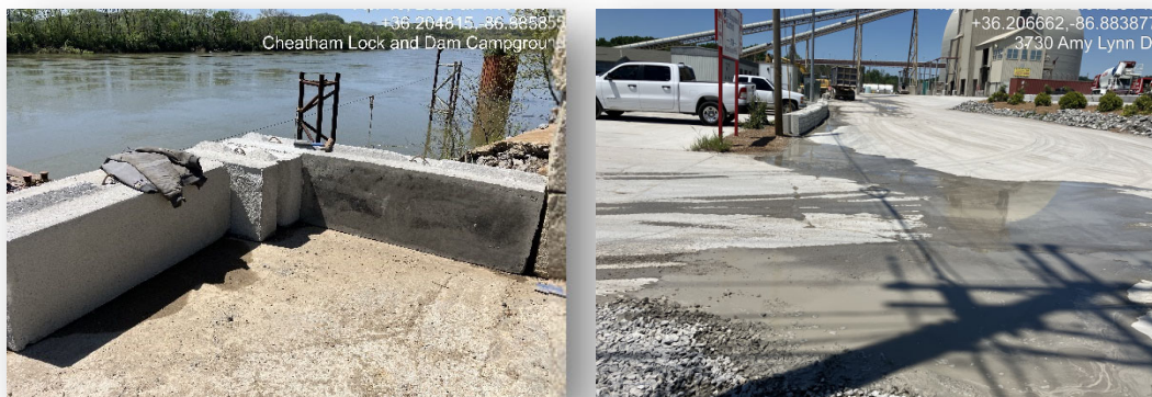
Corrected outfall (left) and Non-Stormwater Discharge (right) at Barge Facility
