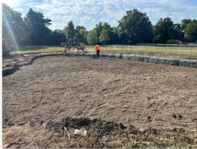
Photo of One of the Infiltration Basins During Construction
