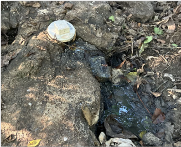
Photos of the Leaking and Repaired Private Sanitary Sewer Service Line
