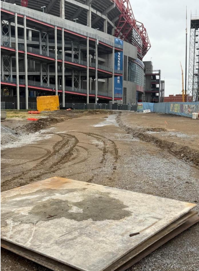
Subgrade and path for the new S. 2nd street
