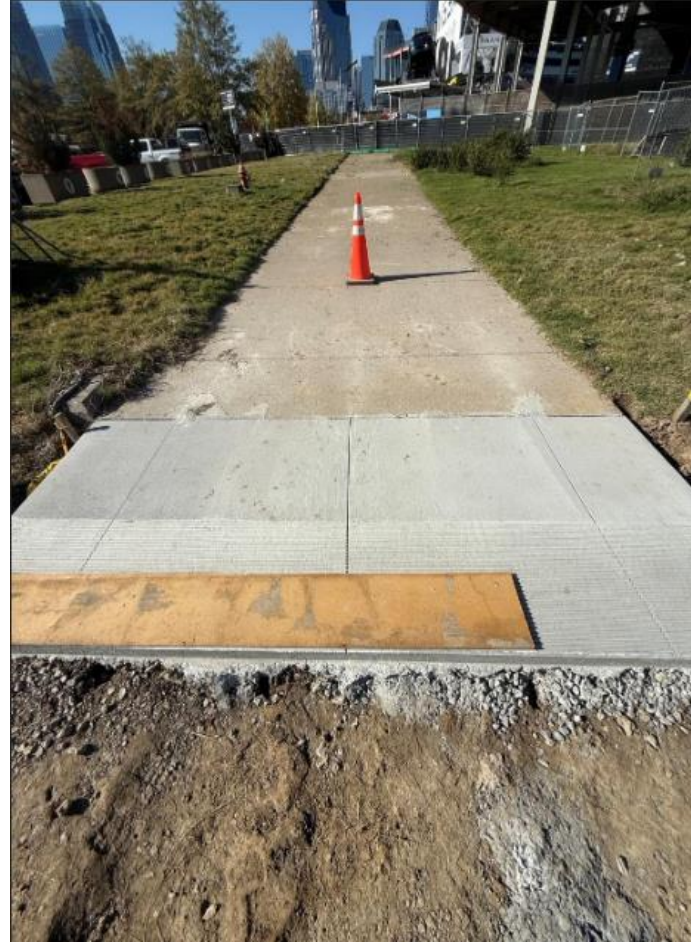
Tactile warning along S. 2 nd street facing West.
