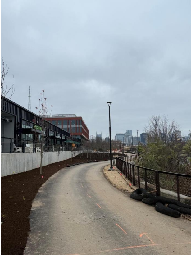
Site lighting and landscaping along the walking path
