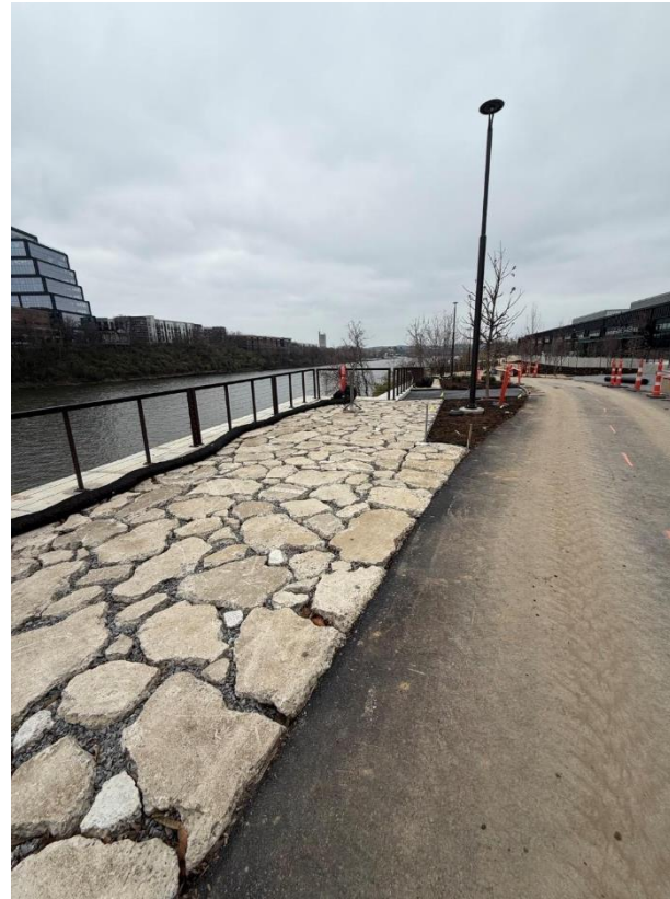
Paver stones and benches built from existing concrete that was removed during demolition
