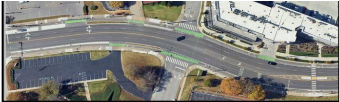
Bike Lanes on 12th Avenue South Featuring Green Pavement Markings at Driveway Crossings and Vegetative Buffers
