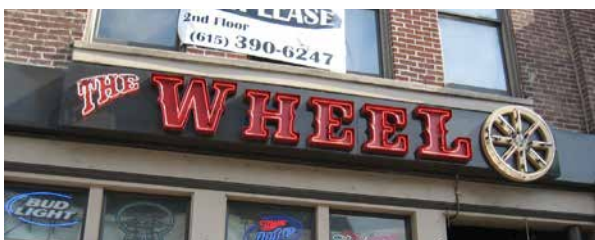
Example of raceway incorporated as sign background
