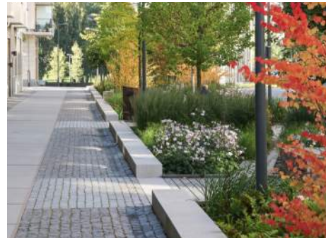
Storm Water Retention Gardens
