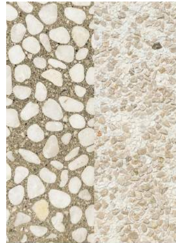
SIDEWALKS & PORCHES exposed aggregate permeable concrete
