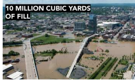
Image of 2010 Flood illustrates the challenge of building in a floodplain
