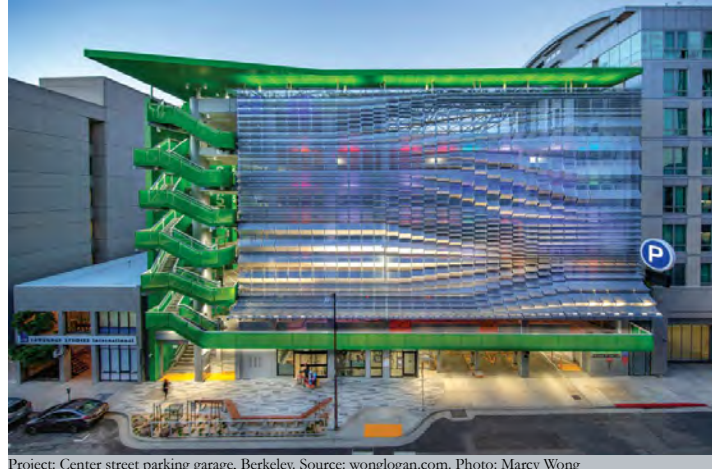
Project: Center street parking garage, Berkeley. Source: wonglogan.com. Photo: Marcy Wong
