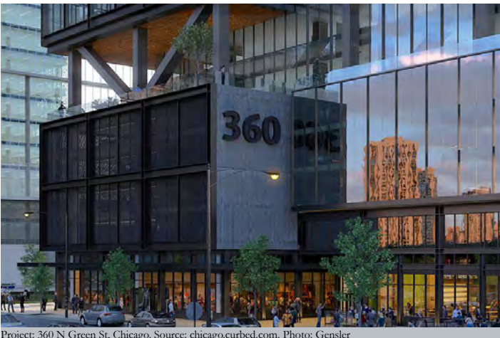
Project: 360 N Green St, Chicago. Source: chicago.curbed.com. Photo: Gensler
