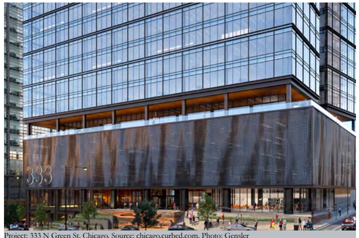
Project: 333 N Green St, Chicago. Source: chicago.curbed.com. Photo: Gensler
