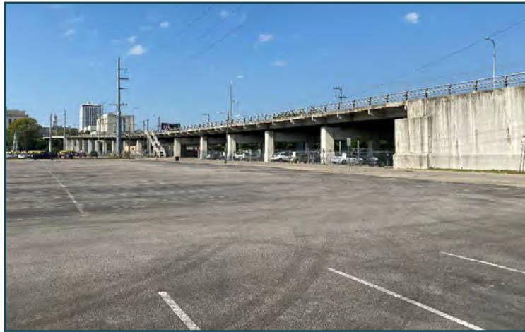
James Robertson Bridge Existing Condition
