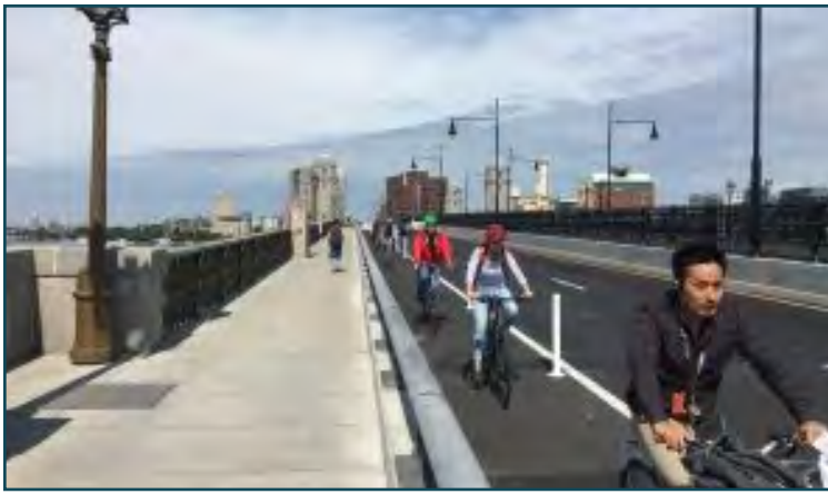
Example of bridge restriping and expansion for enhanced bike/ped facilities
